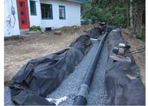
Cyane Gresham's garden – drainage installation
